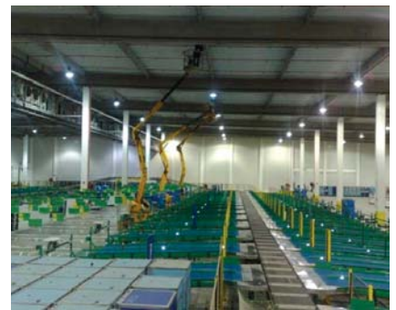
➤ Metrolight's Solution Installation
