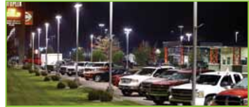
After Metrolight 450w EcoBOX Retrofit solution - matching light levels!
