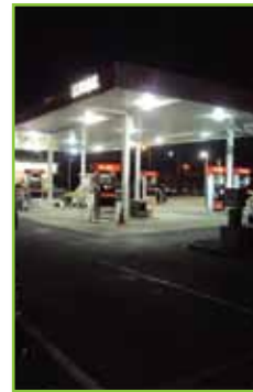
Before Metrolight 320w magnetic HID ballasts
