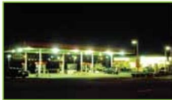
Before Metrolight 320w magnetic HID ballasts
