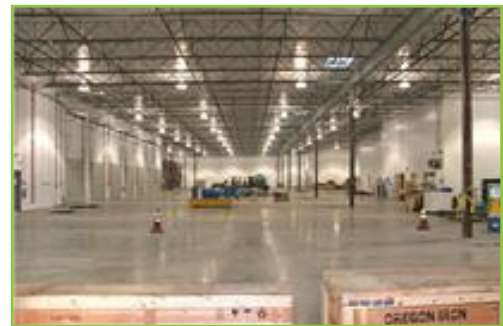
After Dimming 450w Retrofit Kit Solution with New Reflectors
