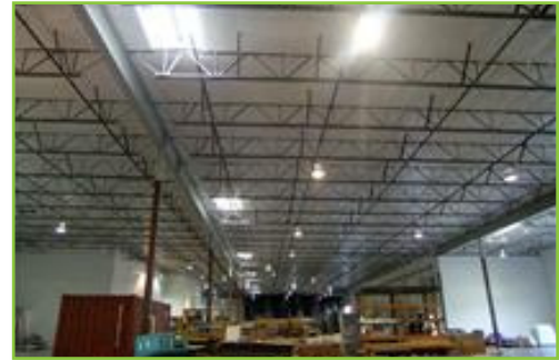
Before Dimming 400w and 1000w Metal Halide High Bays
