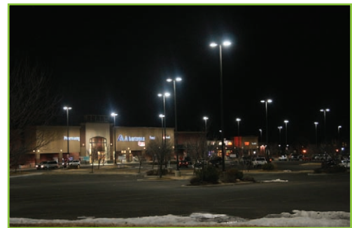
After Dimming 400W SmartHID™ Retrofit solution. Maintained lumen levels while reducing lamp power
