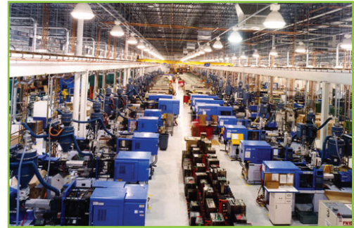
TE Connectivity Previous lighting system at the manufacturing plant
