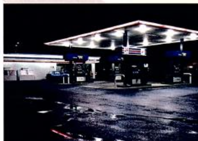
Flying K Gas Station After Metrolight: 250W SmartHID™ Electronic Ballasts – Maintaining Light Levels
