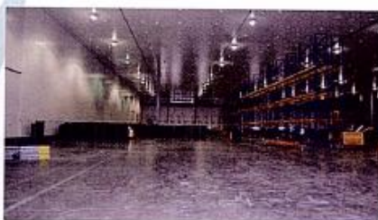
UK Grocer Distribution Center After Metrolight: 350W MH Electronic Ballasts
